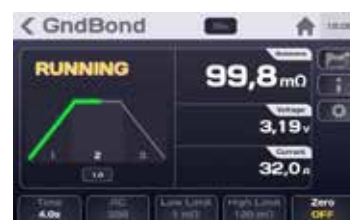
On going test
